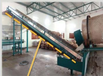
Hopper Delivery Conveyor
